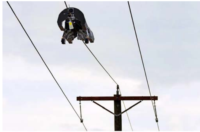
Fig. 6: A Typical Aerial Fibre Optics Installation [38]
